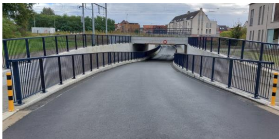
Picture: Finished tunnel at Vossenslag (Herentals)
