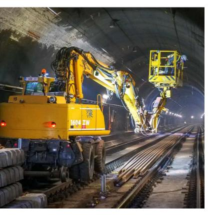
The track specialists therefore made the most of the spring holidays 2019 to replace numerous components at *Liège-Carré*, such as rails, sleepers and ballast. In the tunnels on this section of the L34 *Liège-Liers*, the catenary technicians have also started the preparatory works for the renewal of the power supply device.
