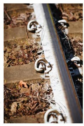
The painted parts belonged to "higher risk" zones, such as metal bridges, which are even hotter and accelerate the deformation of rails. The curves were also painted white, as they offer less effective resistance to the traction exerted by the expanding metal.
